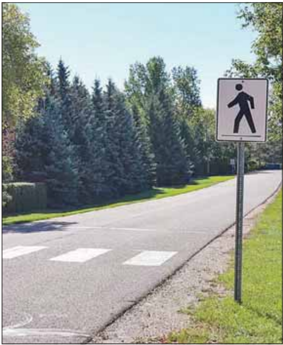
New crosswalk TOWN OF WHITE CITY | GRASSLANDS NEWS Pedestrians and drivers in White City will notice a change on Galloway Street this week after a new crosswalk was installed just ahead of the school zone at École White City School.
