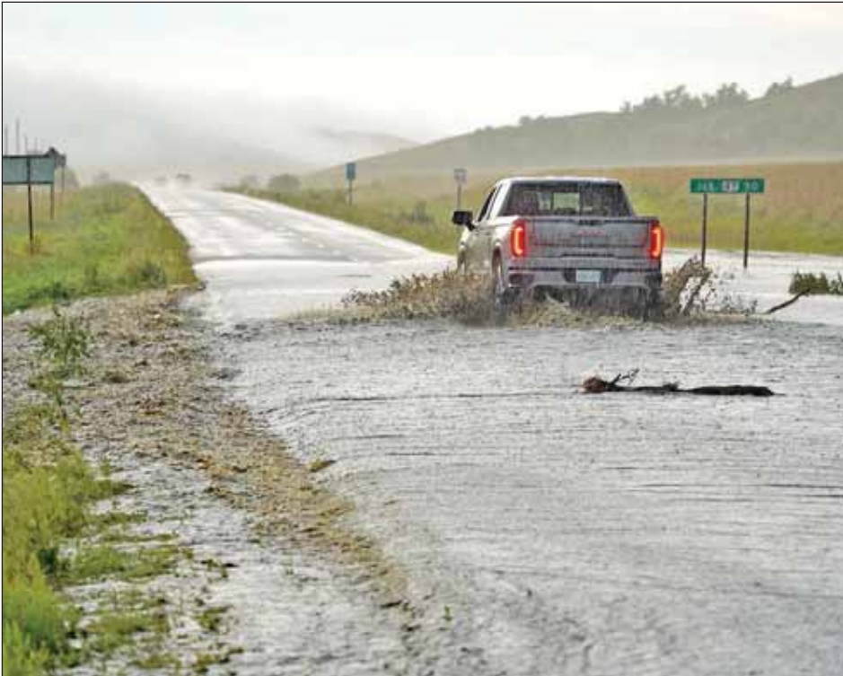
Highways flooded A truck drives through water running over Highway 247 in the Qu'Appelle Valley. The valley saw upwards of 5.5 inches of rain which caused both Highway 247 and Highway 9 in the valley to flood with water running over them.
