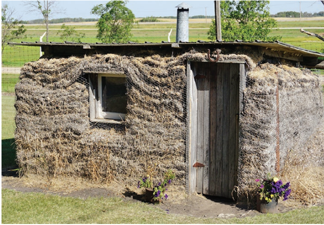
The Broadview Historical Museum's oldest and first exhibit is a reconstructed sod house.
